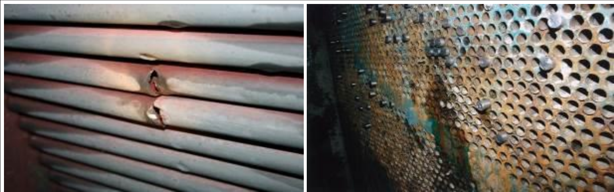
Fig. 1. Defects of tube systems during their operation in NPP condensers
